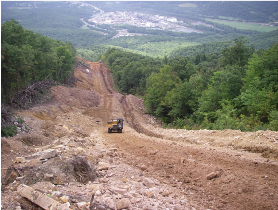
Figure 4 – Example of construction road with adjacent pipeline trench. Material excavated for the road is piled on uphill side of road; material excavated for the trench is piled in a berm on downhill side of trench.
