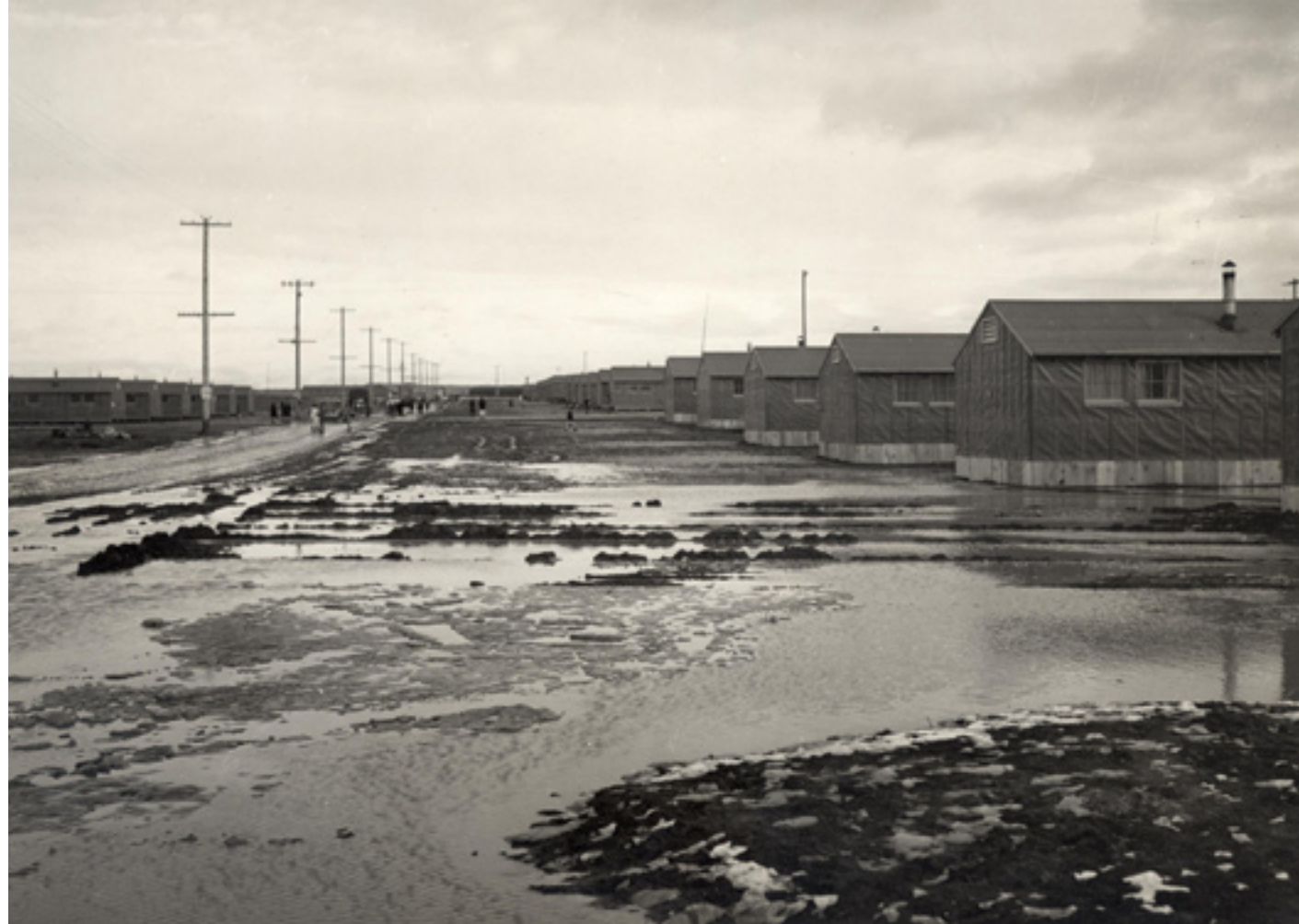
Minidoka Relocation Center, December 1942
