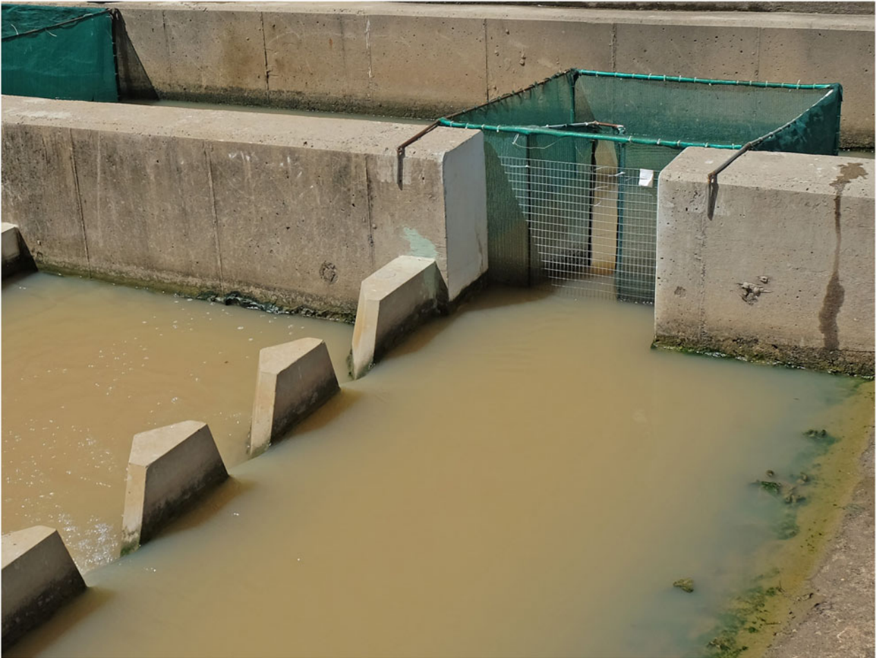
Figure 3. Trap like those used in the case studies, showing small mesh size and large fish exclusion mesh.
