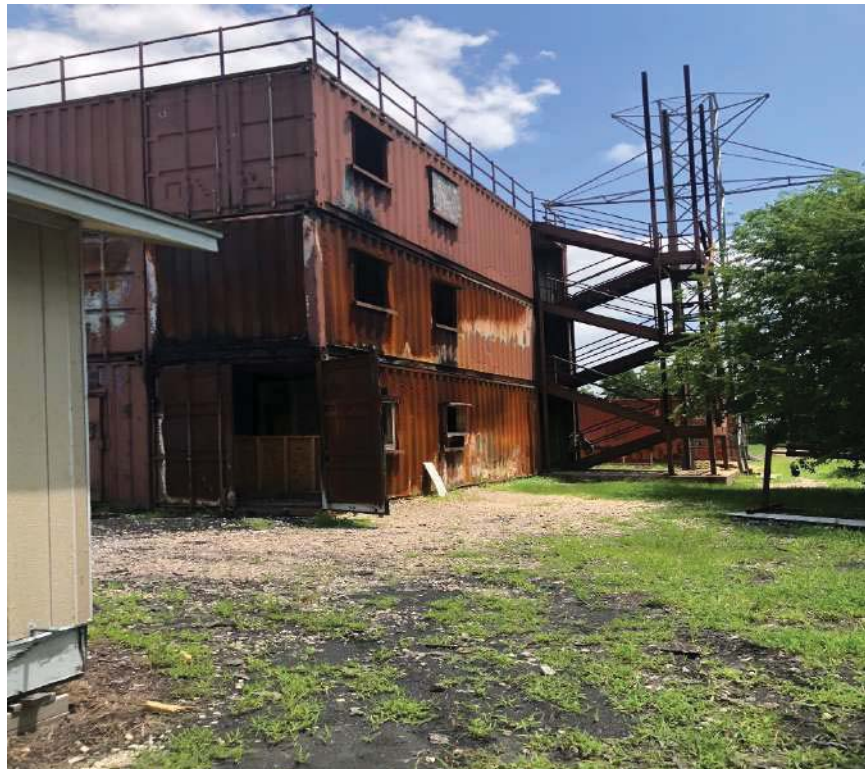
Photograph 6. View facing east away from the Subject Property
