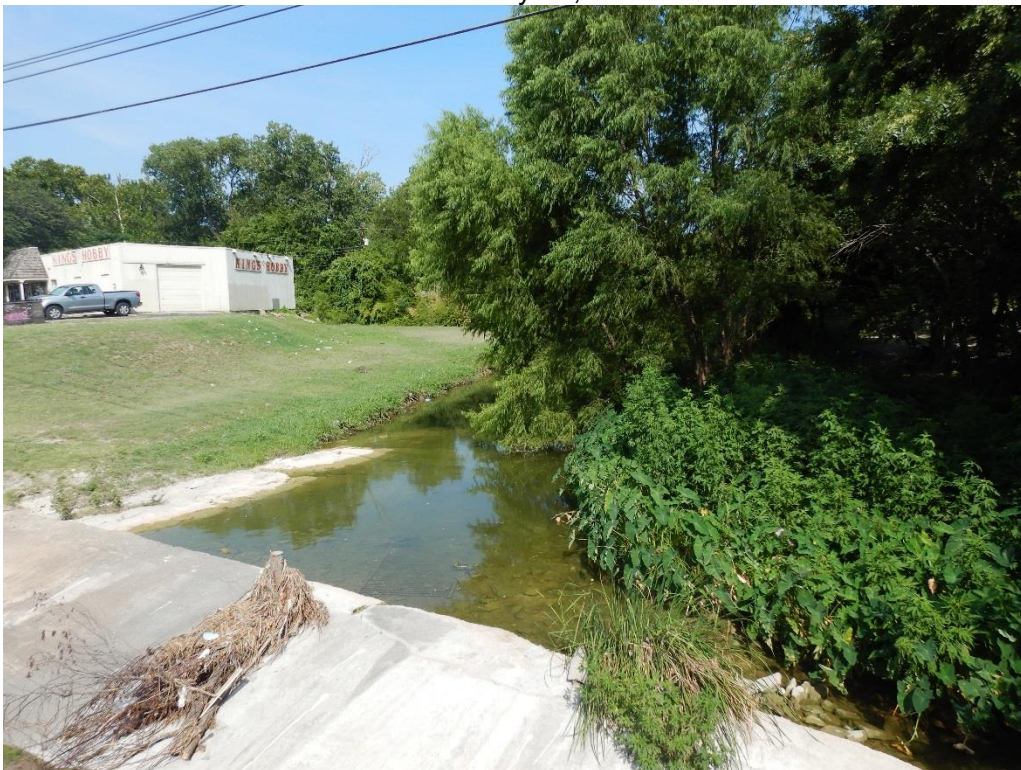
View of Little Walnut Creek facing west from bridge on North Lamar Boulevard on July 24, 2018.
