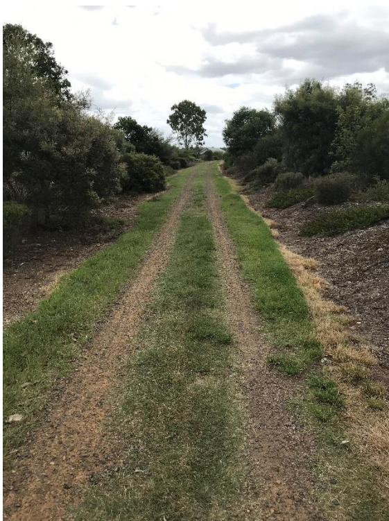
The unpaved section beyond the kilometre of concrete paving
