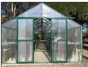
A new Green House was built
