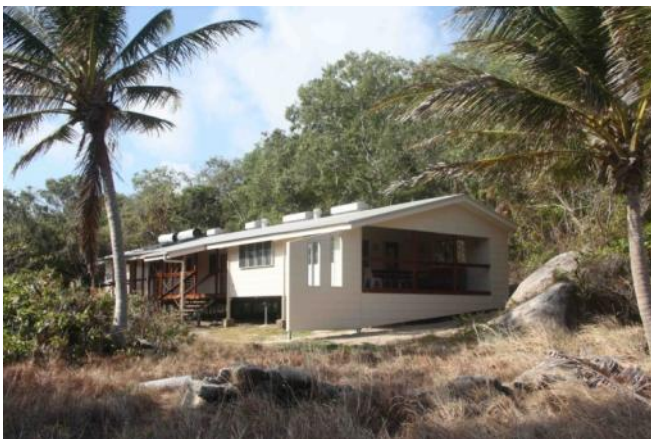
The new Loomis House
