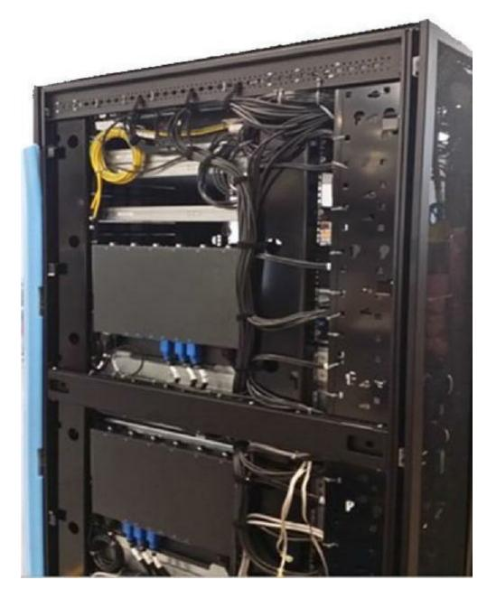
Figure 2-39 Modular 0U PDUs maximize rack space
