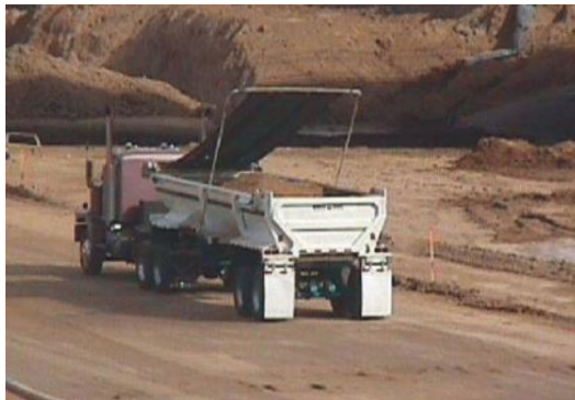
Loaded haul trucks must be covered with tarps to prevent wind blown dust during transport.
