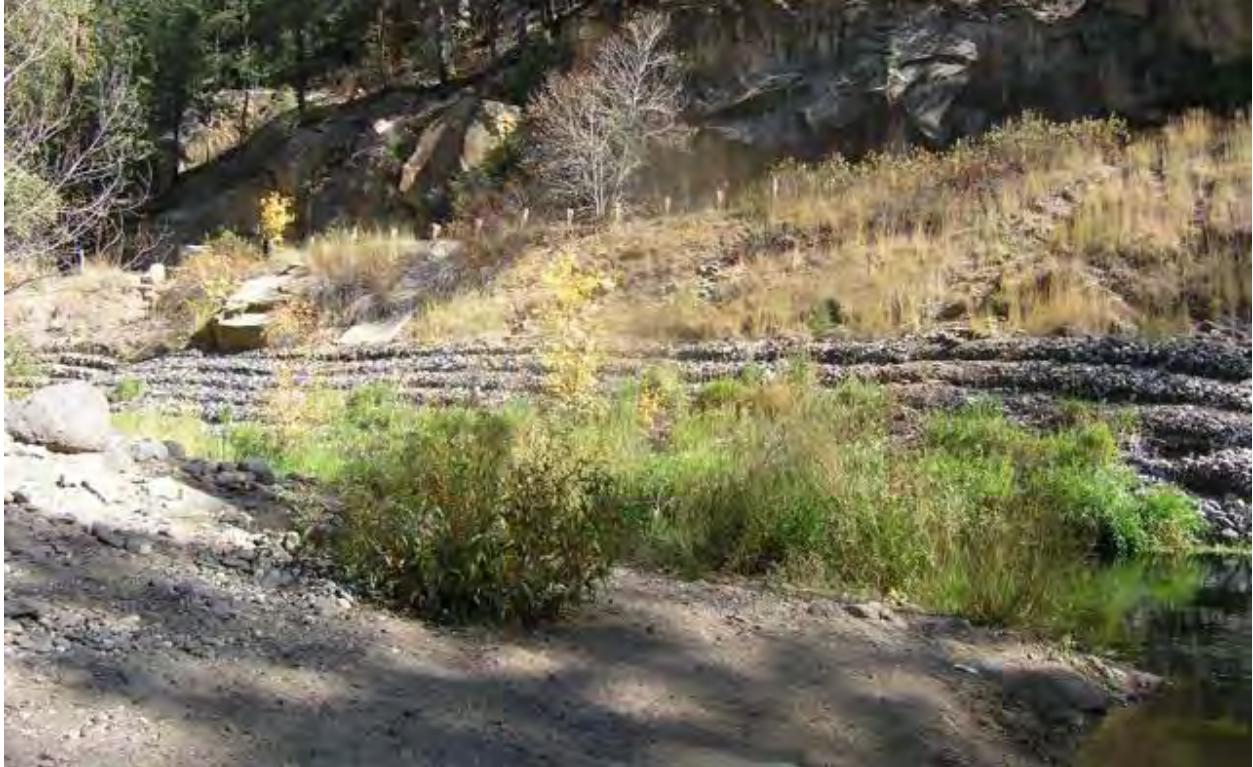
Photo 7. View from the opposite bank of Oak Creek showing all but the lower end of the project area, facing east. Note the relative lack of vegetation on the disturbed slope above the existing gabion structures where new gabion structures will extend to the roadway above.
