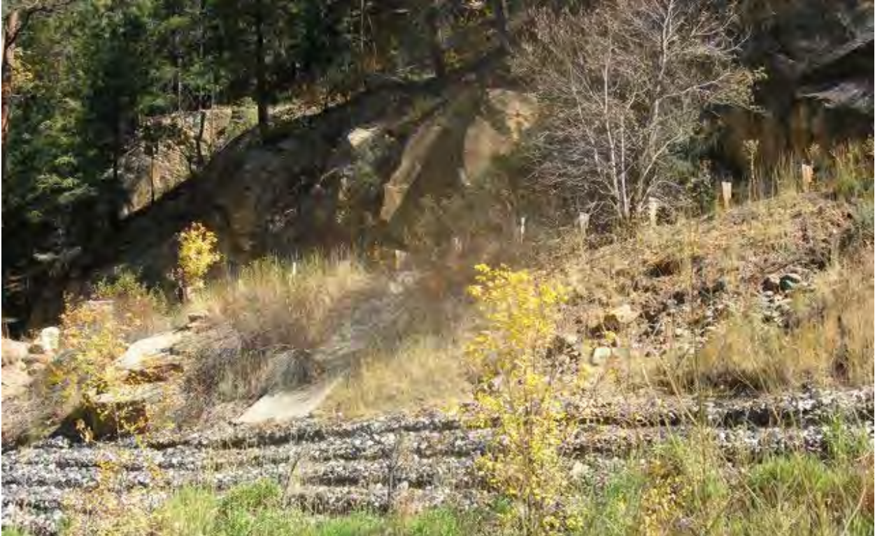
Photo 9. View from the opposite bank of Oak Creek toward the middle of the project area, facing southeast. Note the disturbed slope above the existing gabion structures vegetated only by grasses, low scrubs, and scattered small trees.
