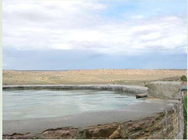
above The restored Wepo Spring catchment basin.
