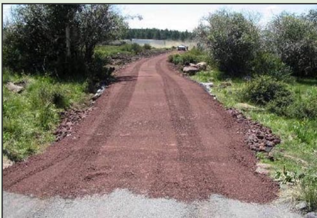
above Meeting of existing permeable fill road (1999) Hart Prairie Preserve, and new road, Fern Mountain Botanical Area, (2008), looking south. Natural Channel Design. Bebb's willow trees on both sides of road.
