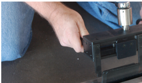
Place Installation/Removal Tool into position onto the Tapers and push them down into the Base Shoe.
