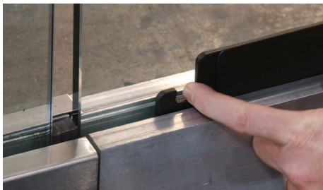
Insert the Taper set half way down into the Base Shoe as shown, opposite the L-Setting Block, and then squeeze the Tapers together finger tight.
