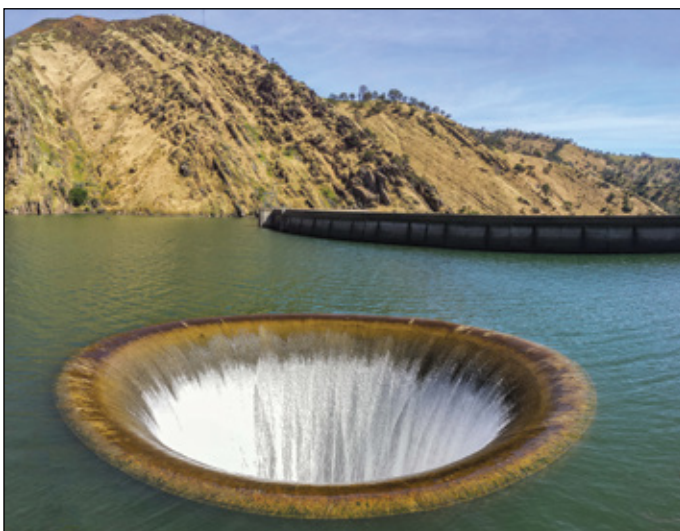
Figure 45. Morning glory spillway at Monticello Dam. Water spills over its lip when the lake reaches 1,602,000 acre feet and a reservoir elevation of 440 feet above sea level. This has occurred about 18 times since 1970, the most recent in February 2019. Although this averages every 2–3 years, it has been common to have 7–13 year gaps with no overflow.
