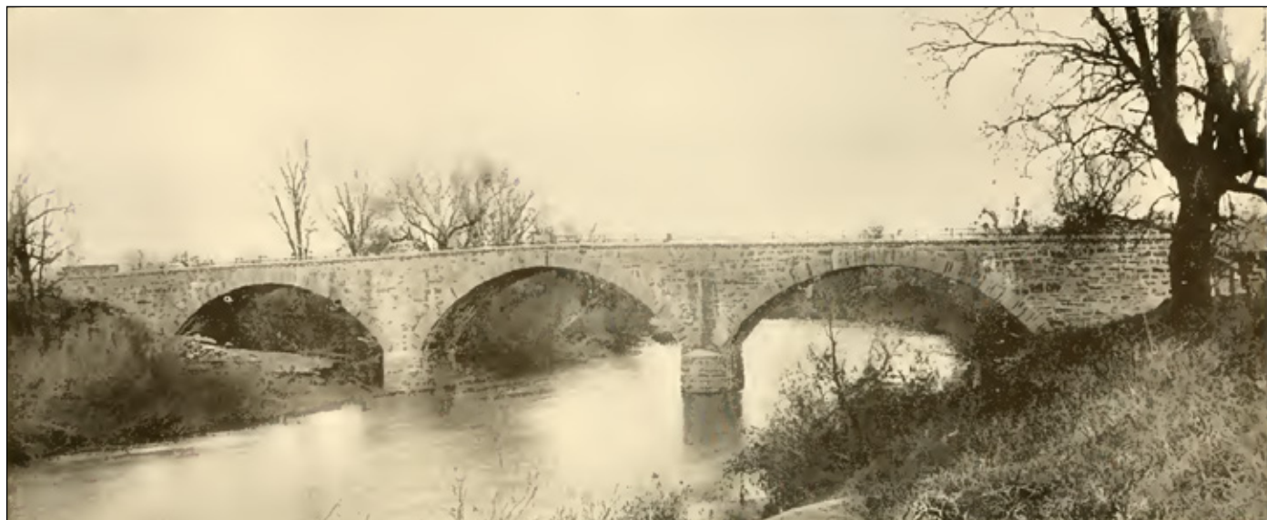
Figure 8. Putah Creek Bridge in Berryessa Valley. Source: Wallace 1901.
