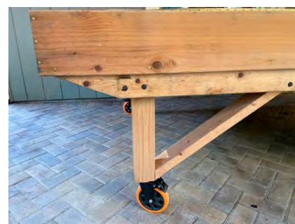
Heavy duty wheels support "box."
