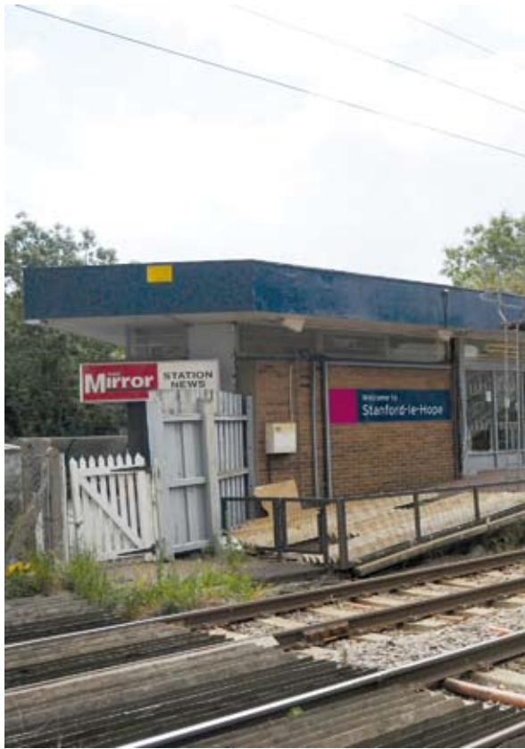
Figure 16 - Stanford-le-Hope railway station
