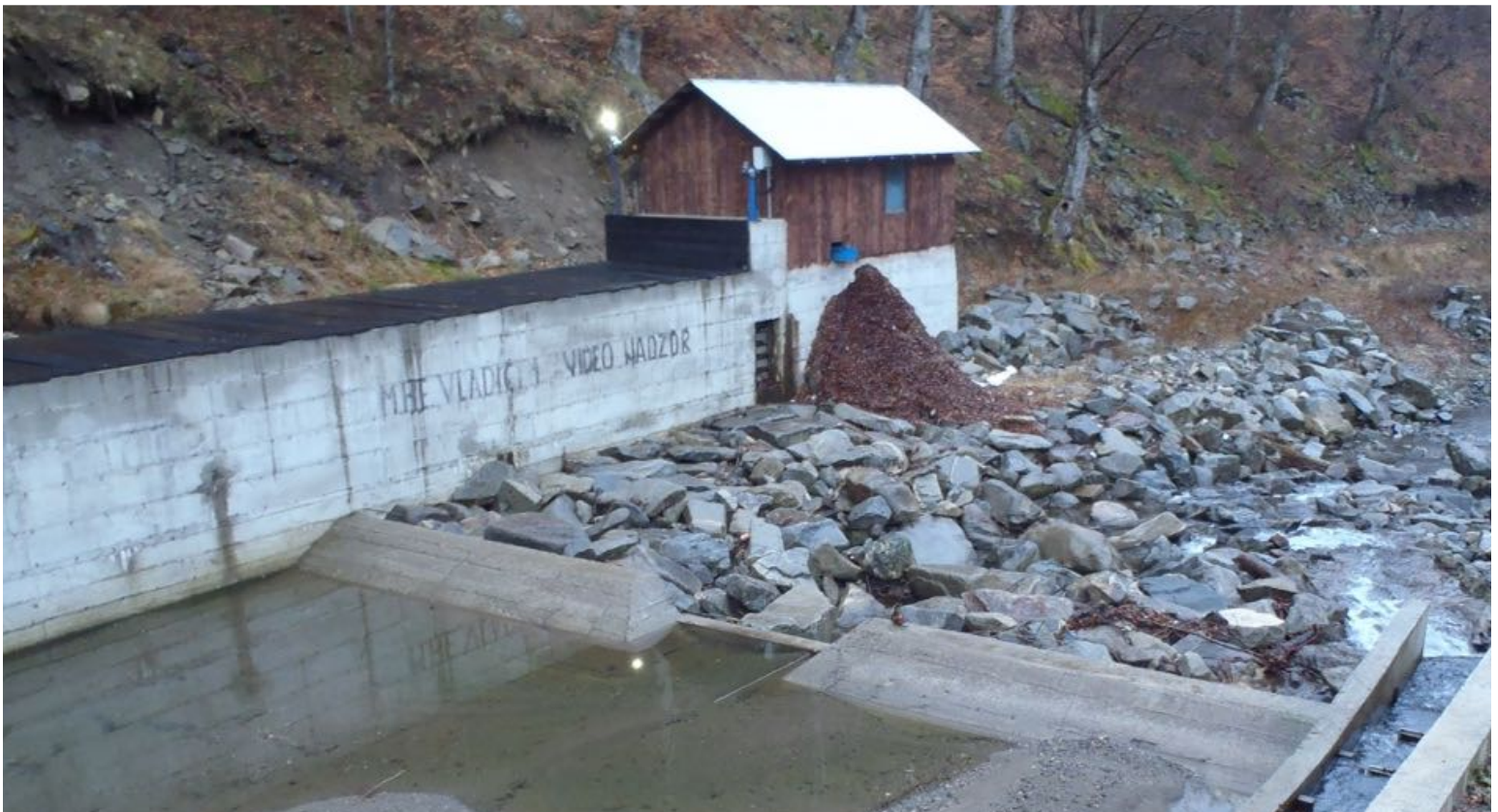
The Vladići 1 plant financed by Erste leaves hardly any water below its intake even in February, let alone summer. Photo: Igor Vejnović
