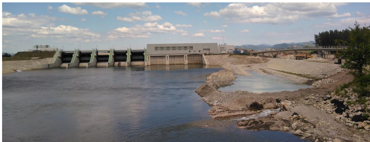
The new EIB-financed Brežice plant on the river Sava in Slovenia. Hydropower projects upstream in Slovenia have exacerbated riverbed erosion downstream in Croatia, lowering groundwater levels. Photo: Pippa Gallop
