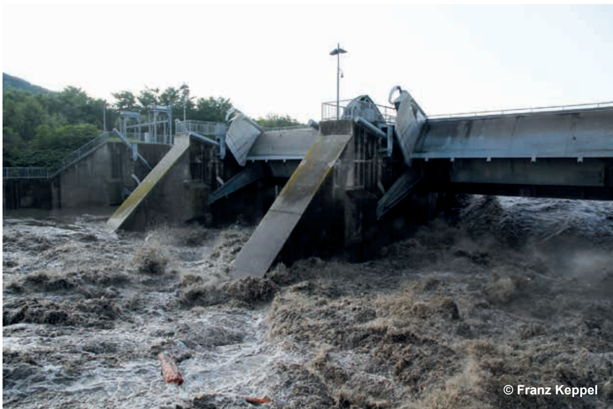
Fig. 3. Example of a run-of-the-river reservoir being flushed on the Mur River north of Graz.
