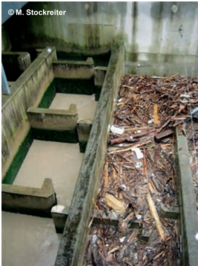
Fig. 11. Debris jam on the vertical-slot pass on the Ill River, at the Hochwuhrl power plant in Voralberg, Austria (BMLFUW2012).
