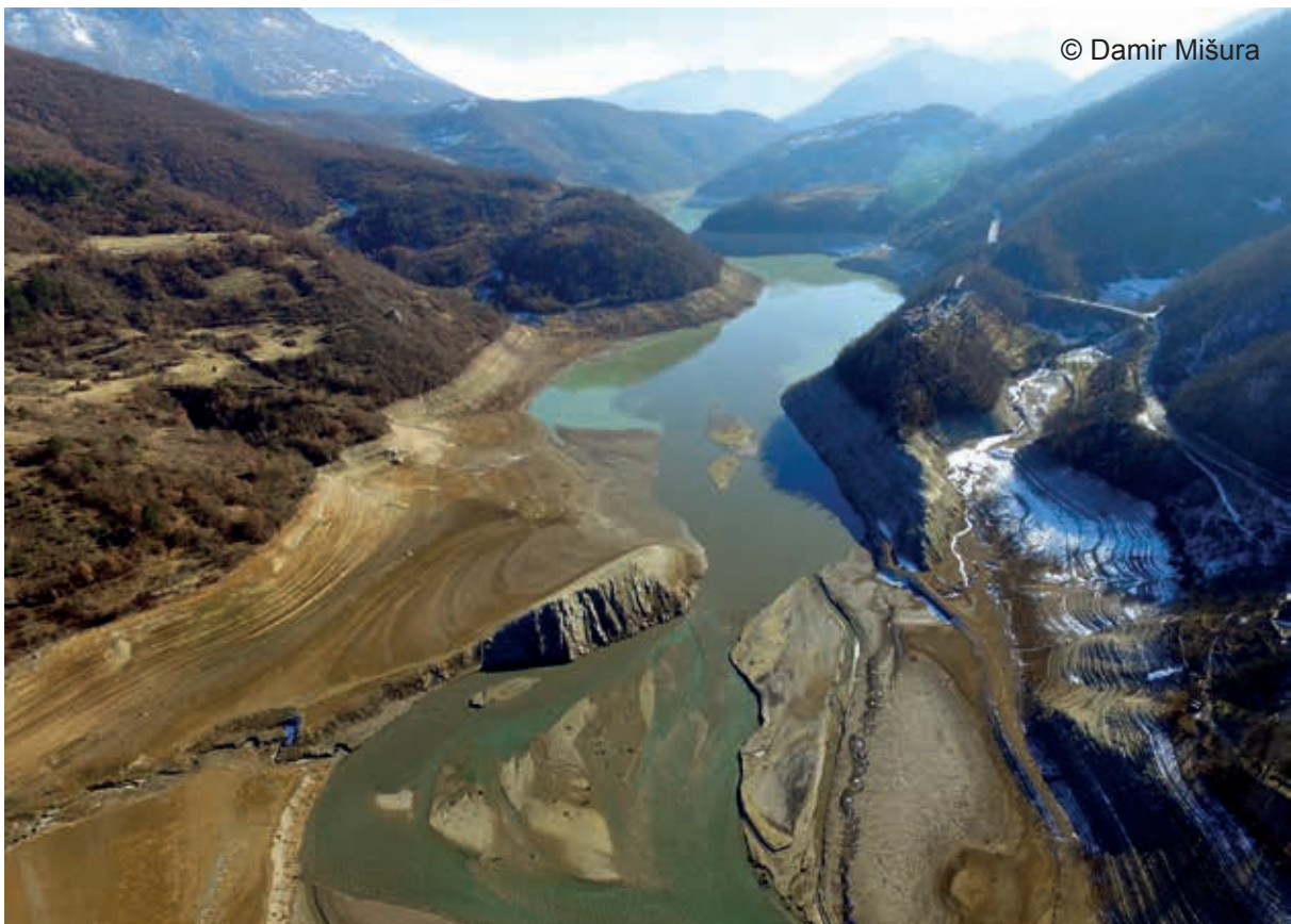
Fig. 6. Aerial view of the Jablaničko Reservoir in early February 2017 after flushing.
