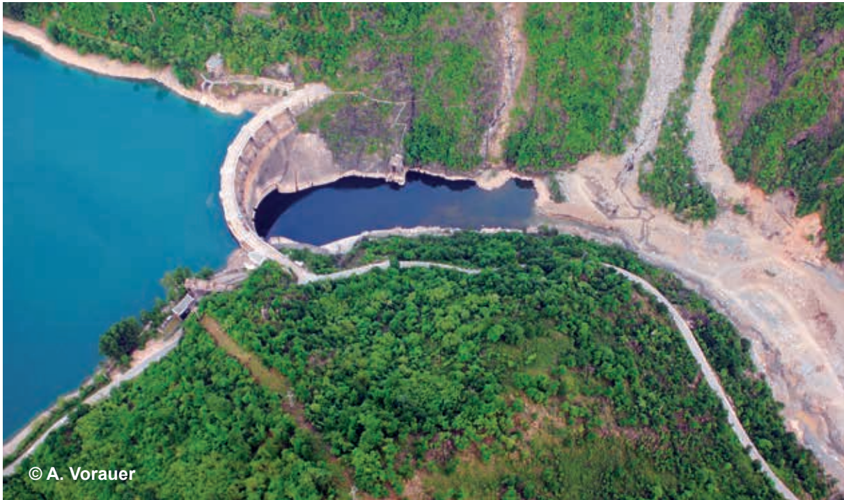
Fig. 9. Storage diversion dam for hydropower generation on the Neretva River, Bosnia-Herzegovina showing no residual flow and a dry river channel below the dam.
