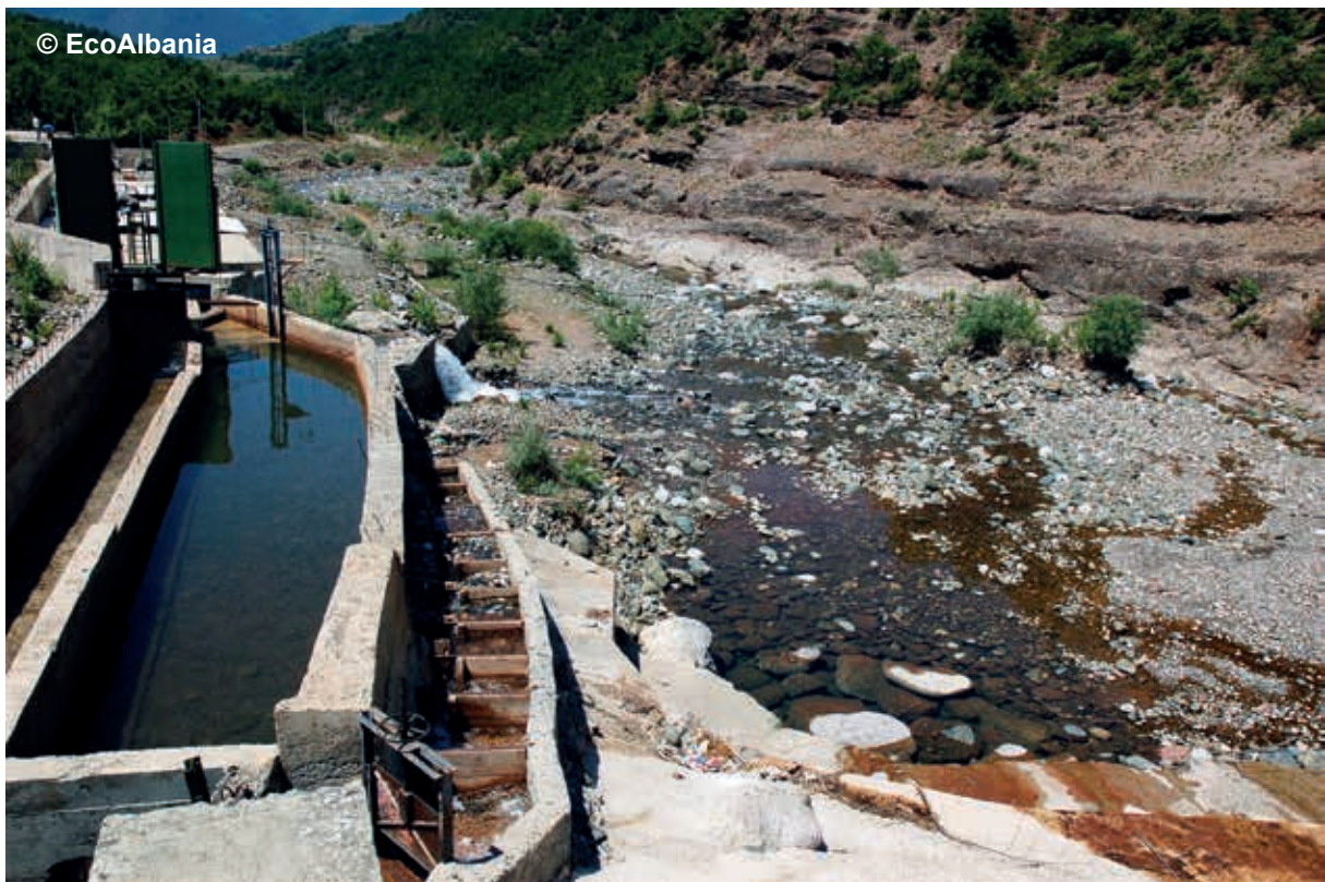
Fig. 8. Power plant on the Rapuni River, Albania. Neither the flow in the fish pass nor the residual flow below the dam is sufficient for sustaining life in the river
