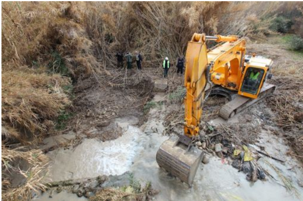
Weir demolition in the Moratalla River
