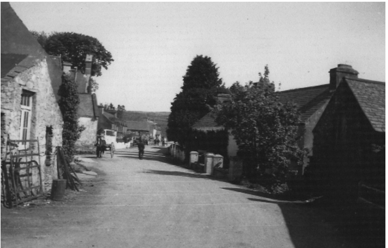
View east through Ballingearry
