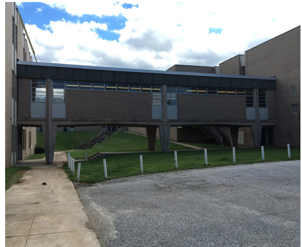
Bridge connecting William C. March to Harford Heights
