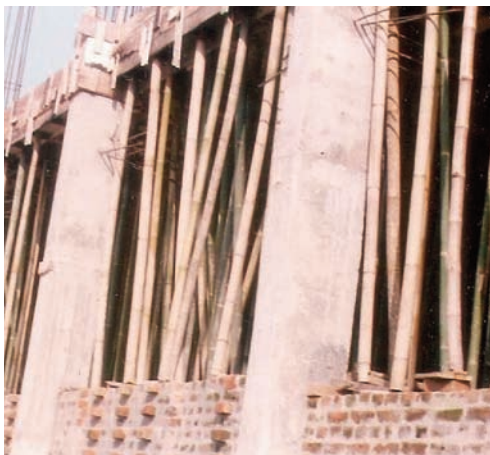
A. Bamboo use as scaffolders
