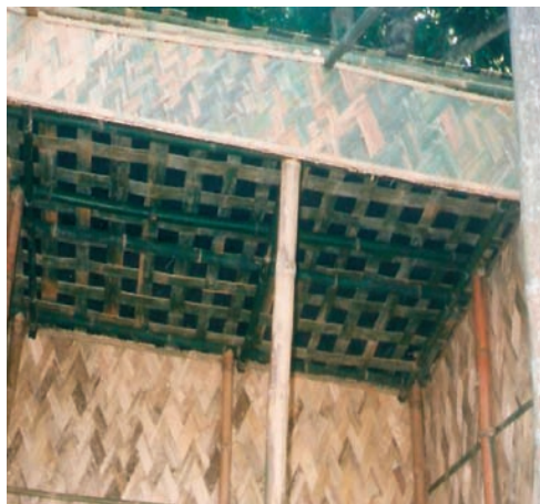
B. Ceiling and wall construction using bamboo
