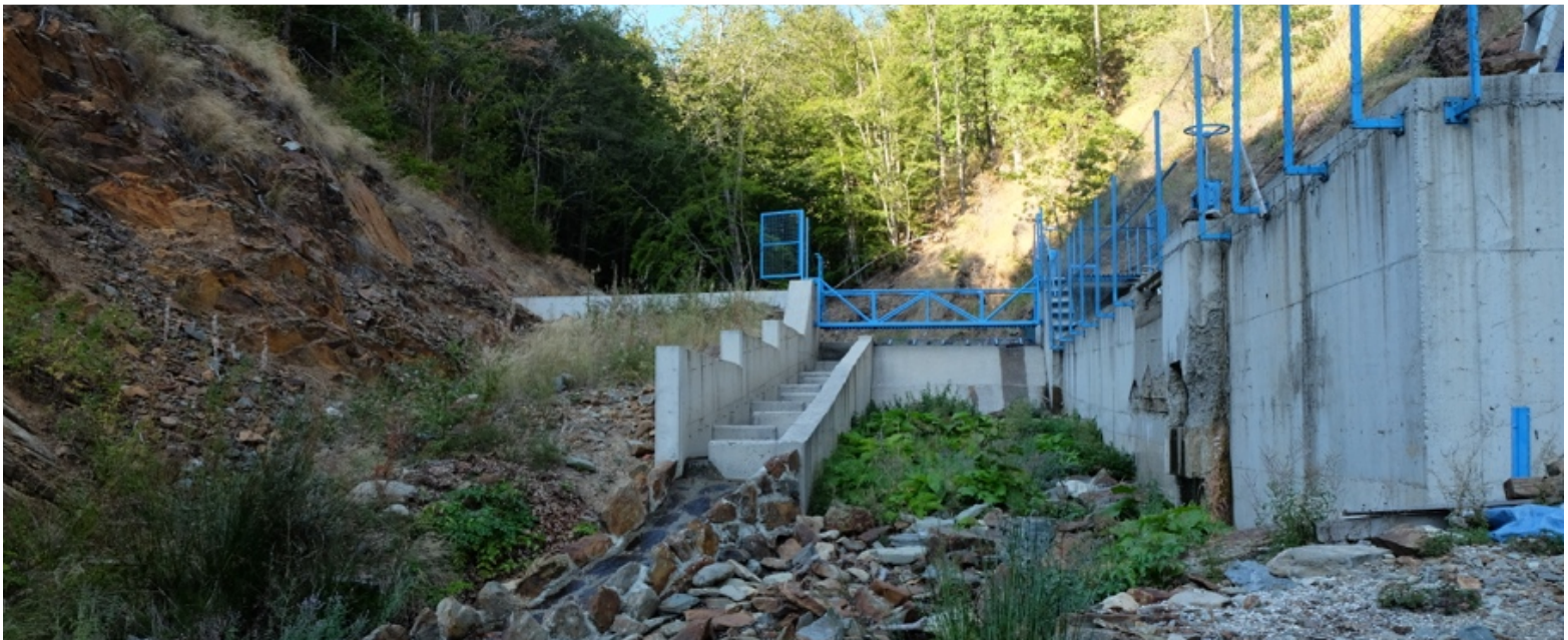
The intake of the Brajcinska reka 1 plant, financed by the EBRD and owned by Feroinvest, is contributing to fragmentation of the habitat of the Prespa Trout. Photo: Igor Vejnović
