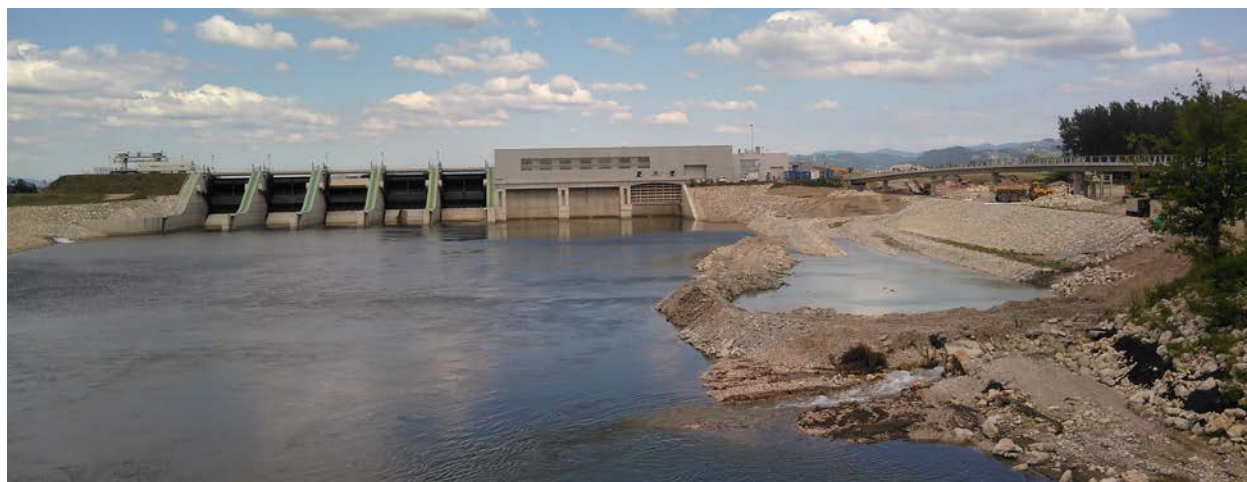
The new EIB-financed Brežice plant on the river Sava in Slovenia. Hydropower projects upstream in Slovenia have exacerbated riverbed erosion downstream in Croatia, lowering groundwater levels. Photo: Pippa Gallop
