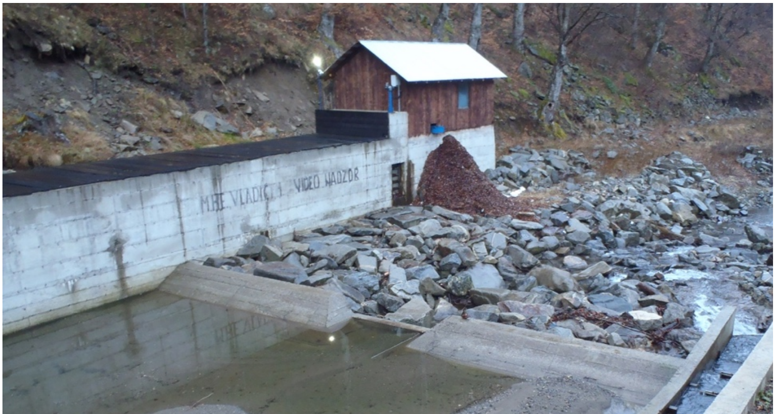
The Vladići 1 plant financed by Erste leaves hardly any water below its intake even in February, let alone summer. Photo: Igor Vejnović
