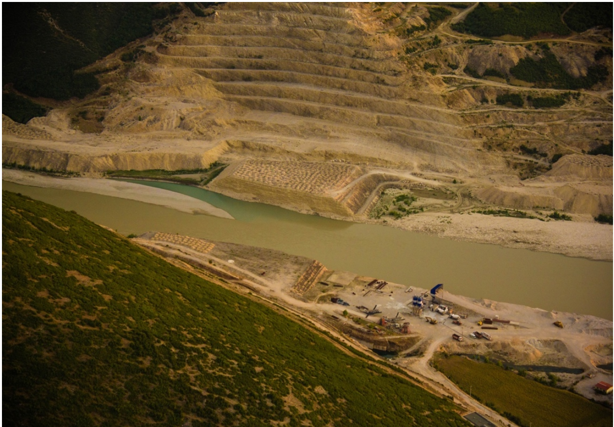
Abandoned construction site of the Kalivac dam on the river Vjosa in Albania. In 2017 a new concession was issued to Turkey's Ayen Enerji & Albania's Fusha to re-start the project. Photo: © Roland Dorozhani
