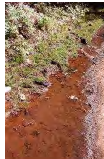
Figure 51. Seep on temporary road on a converted trail surface
