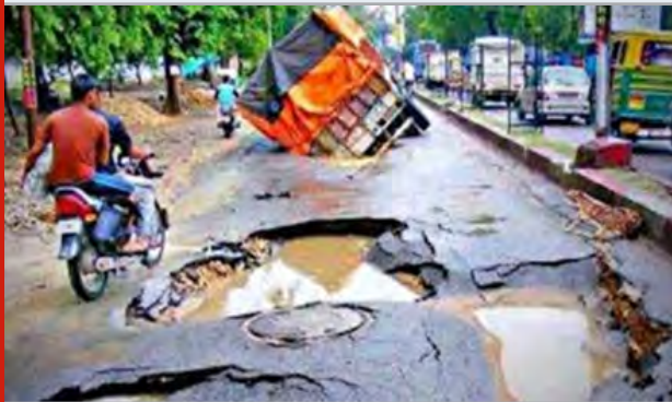
Figure 1: Road accident due to Potholes
