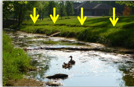
Figure 11: SFG 5.3-UNT 0.1 Tension Crack Bank Failure
