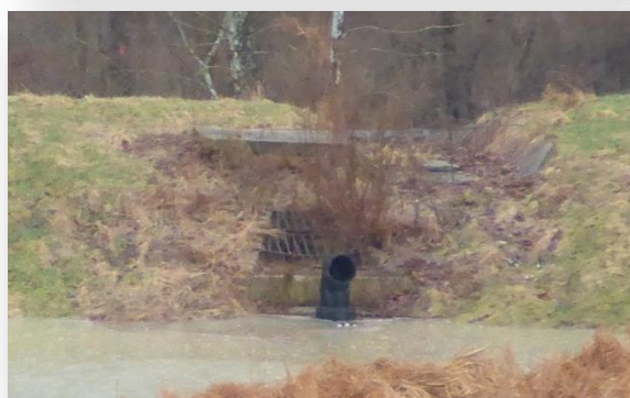
Figure 21: Detention basin retrofit at Northern Kentucky site after installation (top) and detaining stormwater during rain event (bottom)
