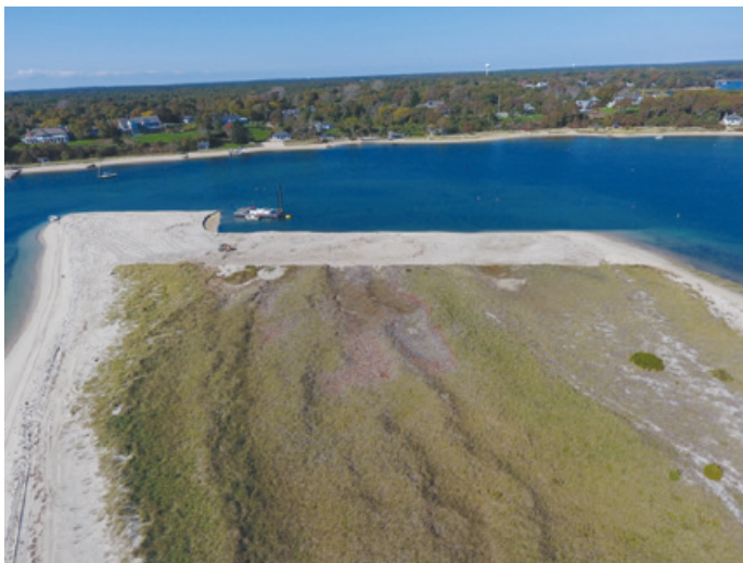
Dredge removes material from western tip.
