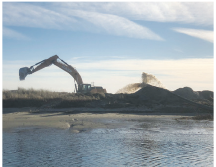
Moving dredged material to the dewatering basin.
