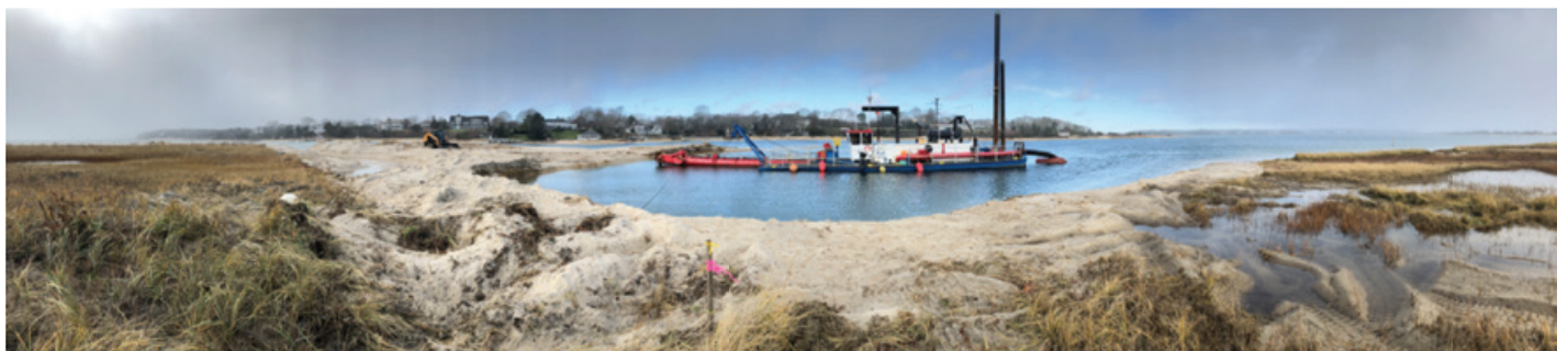
Panoramic view of the dredge in action on the western tip.
