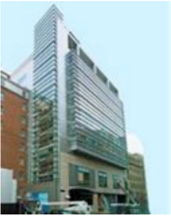
Main South building
