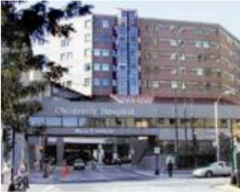
Children's Hospital Main Building front entrance
