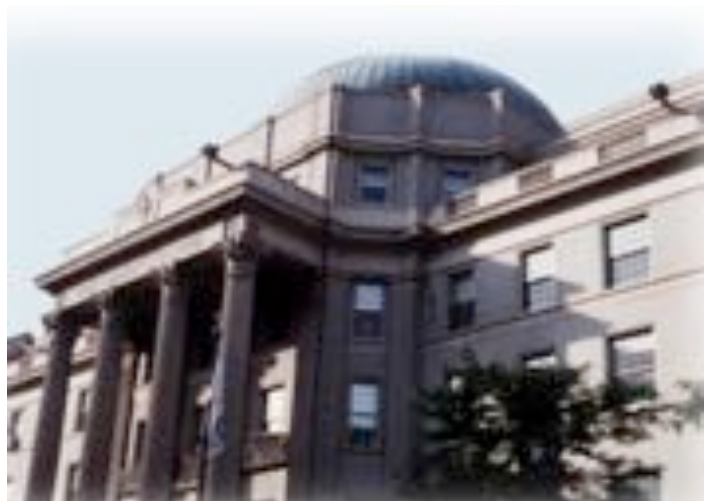
The green-domed Hunnewell building is the architectural signature of Boston Children's
