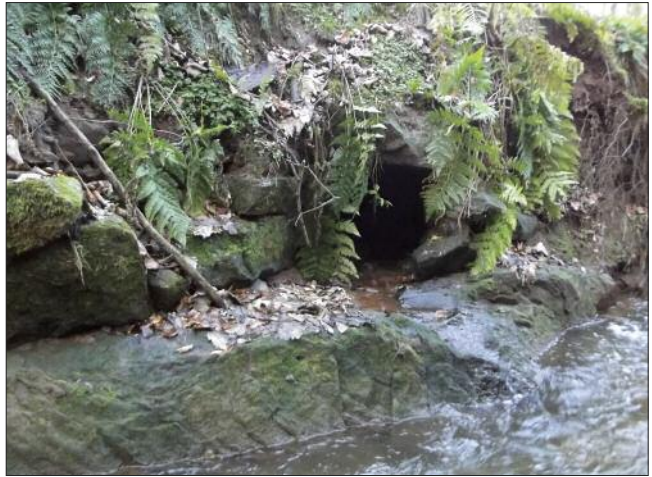
Photo 8. Outflow of culvert with revetment to its left, Dunnottar.
