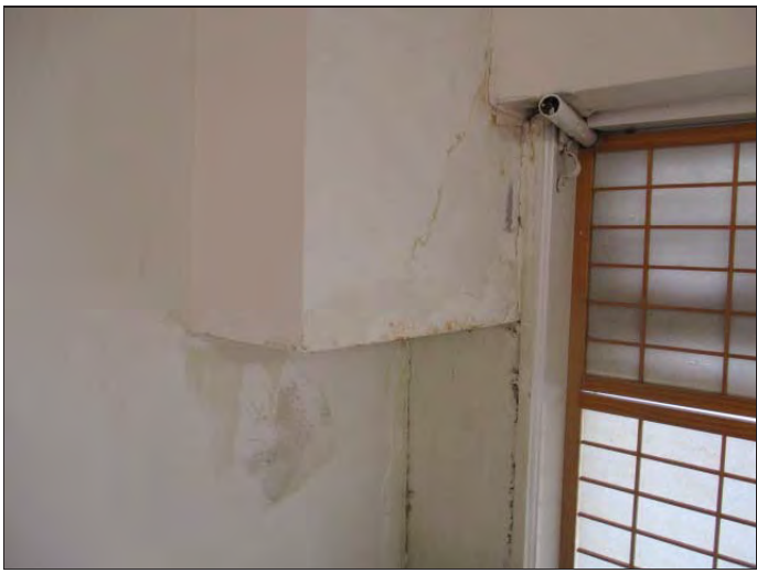
37. Water-damaged wall
