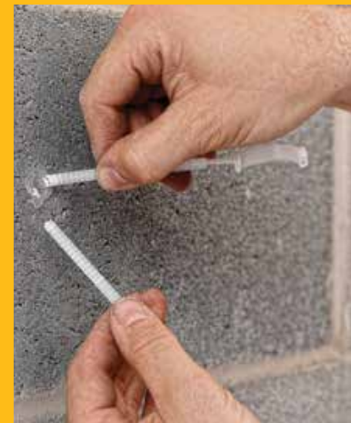
STRAP-TOGGLE INSTALLATION
