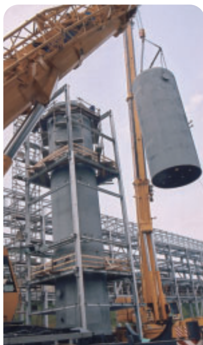
Installing the last element of the oxyhydrochlorination reactor
