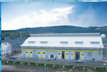
The interior and exterior of the new cell room
