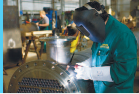
Capital expenditure project of the new chlorine plant in progress in June 2005
