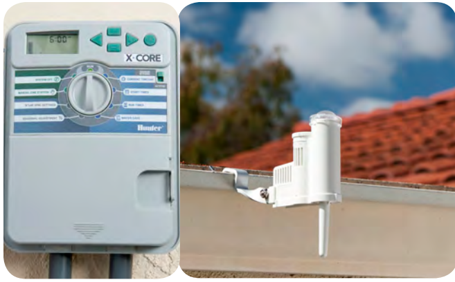
Weather-based controllers often have a sensor that should be mounted outside, free of obstructions, and connected to the controller.
