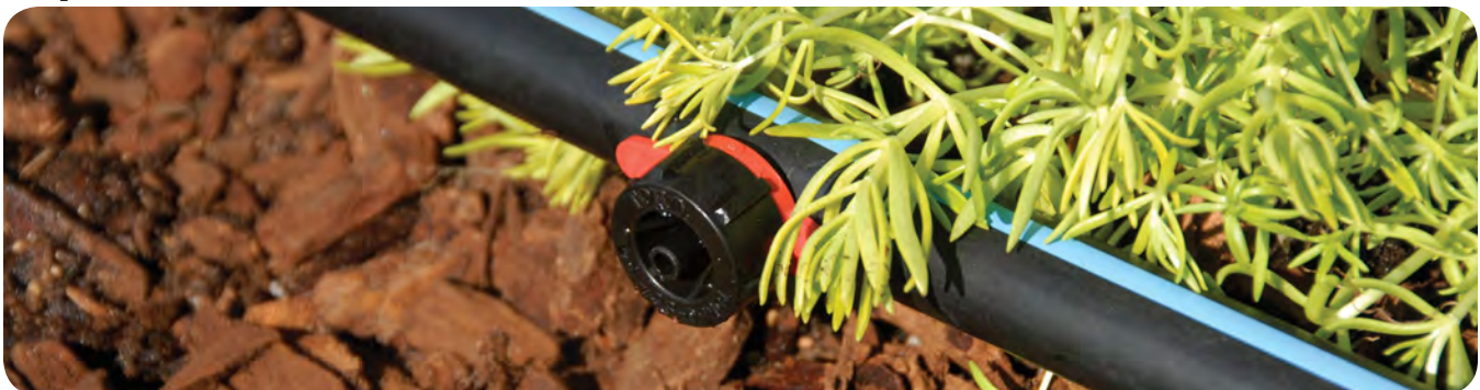
Drip irrigation can be installed at soil surface.
