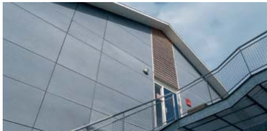
Dansk Eternit Holding produces flat fibre cement sheets used as façade cladding.
