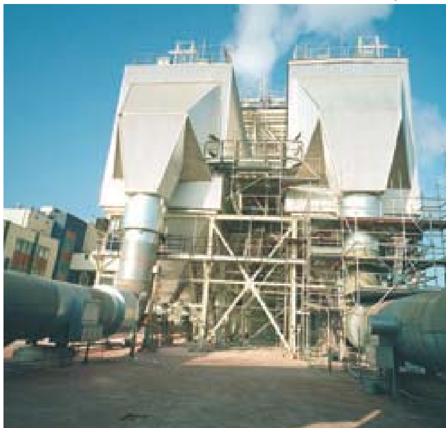
Two electrostatic precipitators supplied by F.L.Smidth Airtech to Nedmag in Holland.
