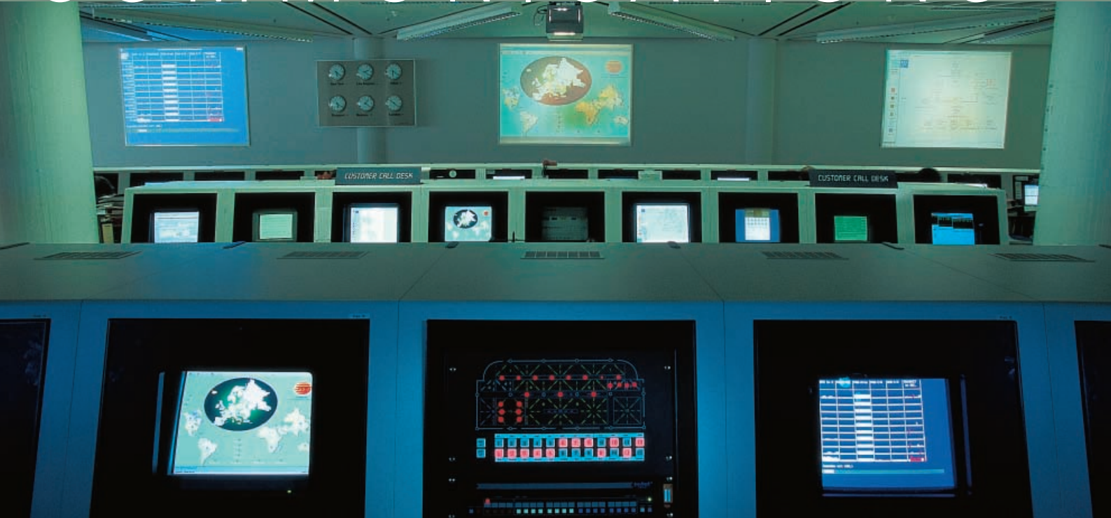
The SBS Command and Control Center registers all incoming customer inquiries and forwards them to the appropriate support staff.
