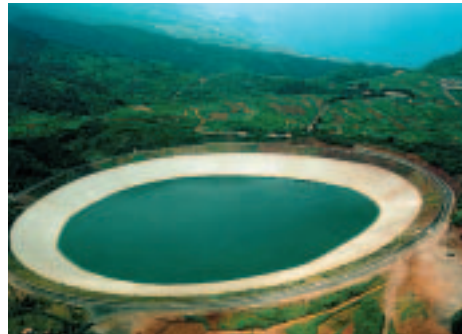
Reservoir at Barlovento (Canary Islands). Created in a volcanic crater with 250,000 m 2 of PVC geomembranes, this reservoir serves to irrigate banana and other food plantations.
