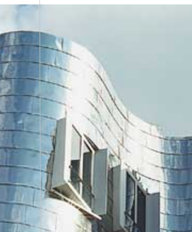
Example of the use of stainless steel: Zollhof in Düsseldorf, Germany
