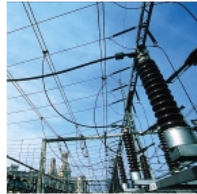
Hydro-electric plant in Central Puerto (Argentina).
