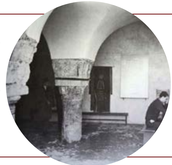
Marble pillars in the Ramban's Shul
