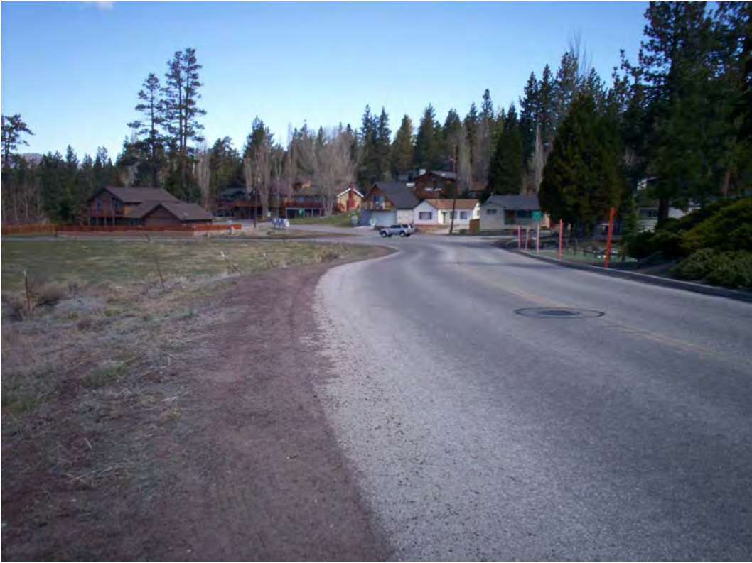
Photograph #9: Residential land use and Moonridge Road east of the site.
