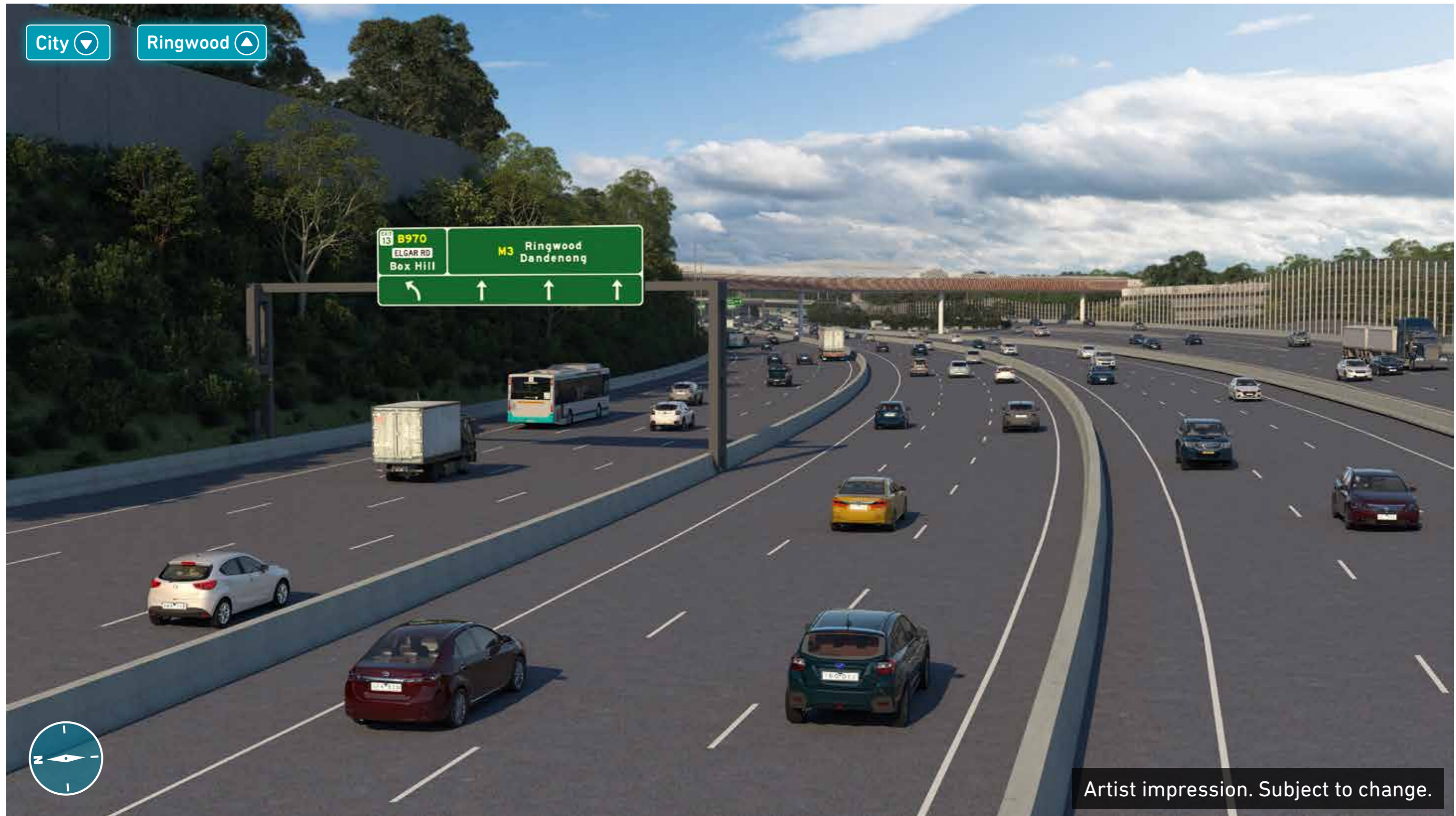
Separated express lanes in the centre of the Eastern Freeway to ease congestion caused by merging and weaving.
