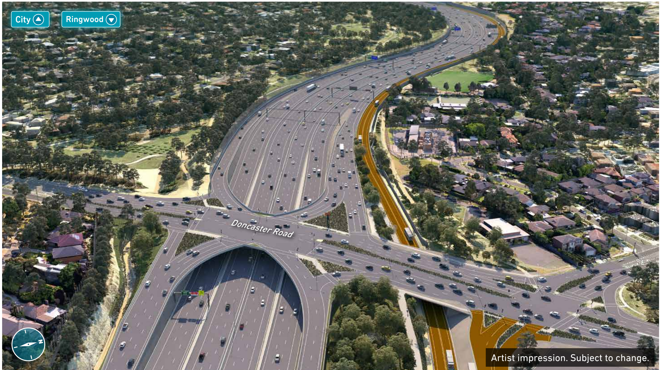
Rebuilt Doncaster Road bridge, new Doncaster Busway and upgraded Eastern Freeway.
