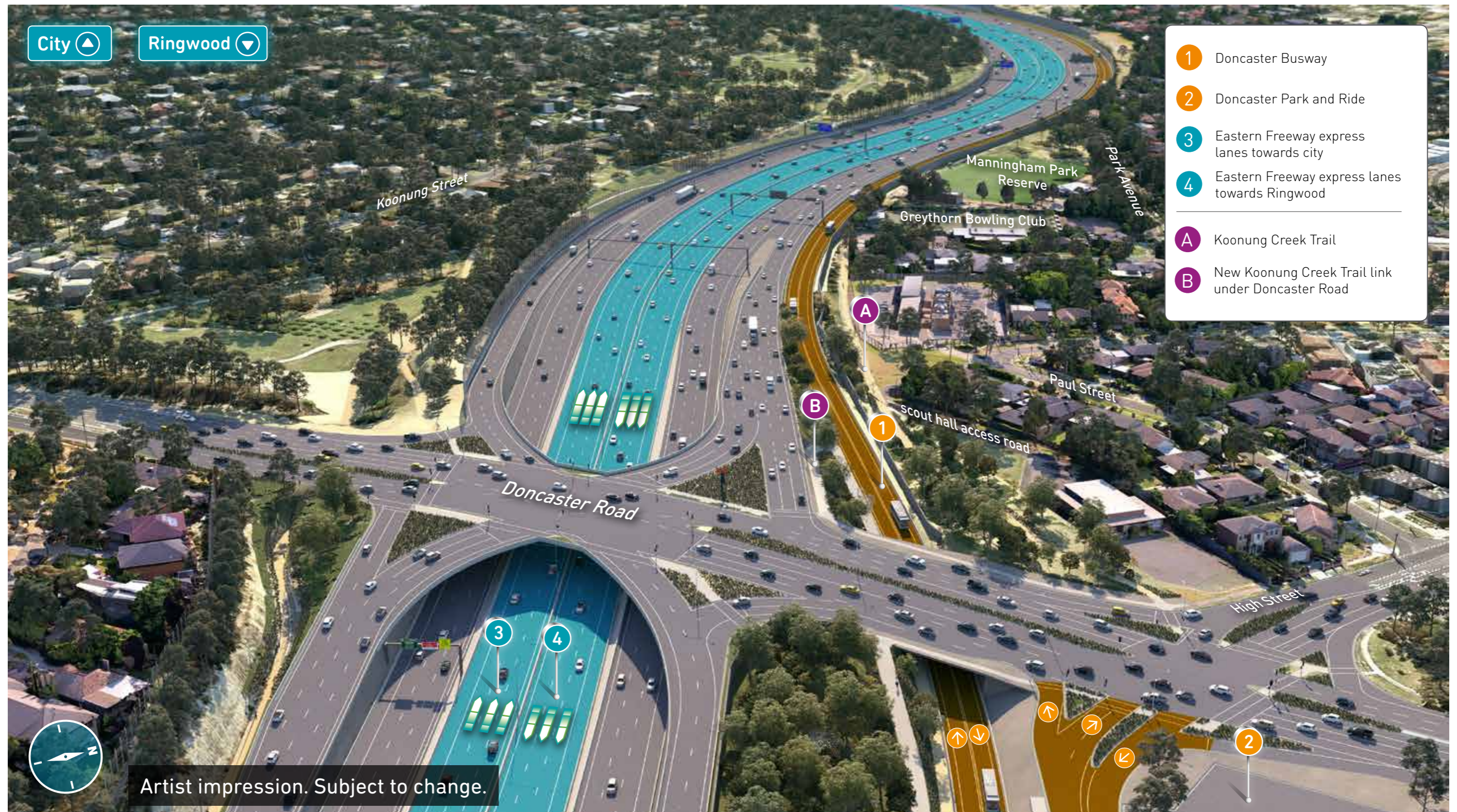
Doncaster Busway and new Koonung Creek Trail link passing under Doncaster Road.
