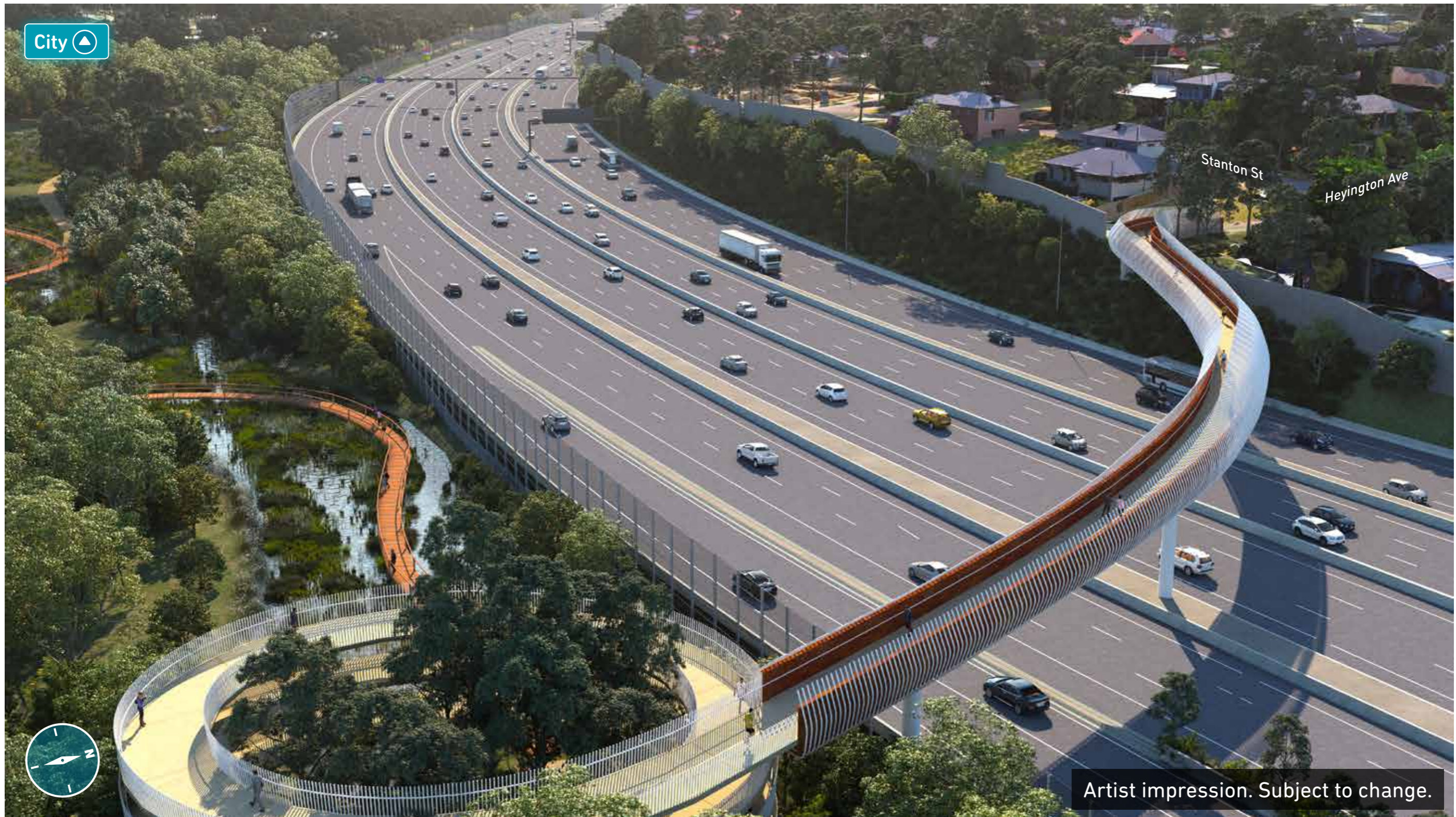
New Disability Discrimination Act compliant walking and bike riding bridge connecting to the wetlands.
