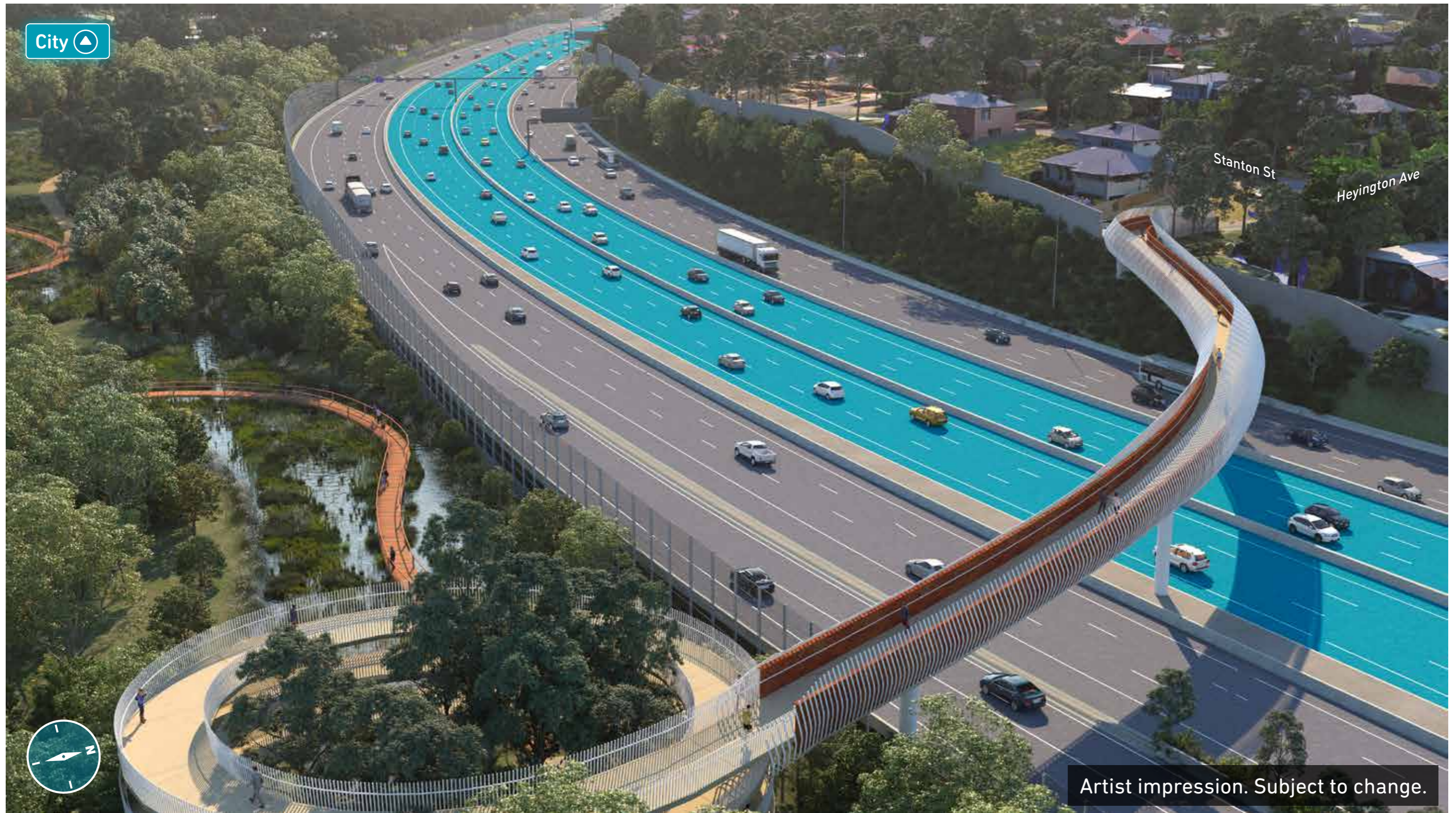
Separated express lanes in the centre of the Eastern Freeway to ease congestion caused by merging and weaving.
