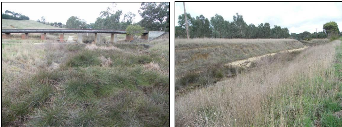
Site 39. Greenhill Creek at Western Highway – north (left) and south (right).
