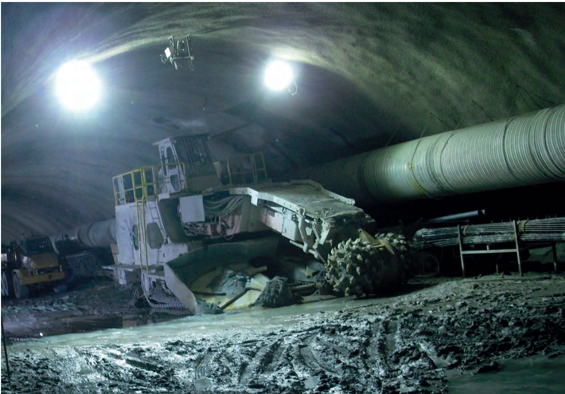
Figure 8-29 Roadheader (Airport Link, Brisbane, 2010)
