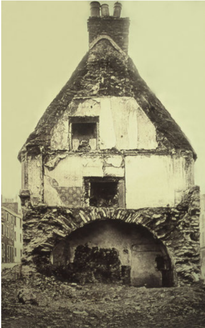
Plate 120. Photograph of a town house in Mid Row, Hawick being demolished. Almost certainly an urban bastle house. Hawick Museum.
