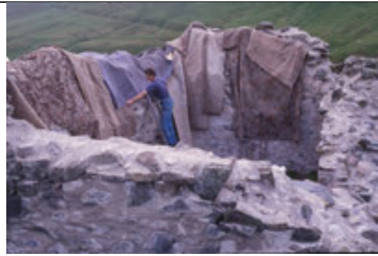
Plate 114. Lime mortar covered for three months.
