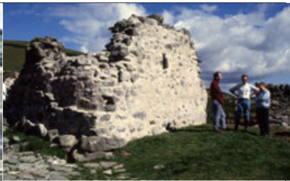
Plate 116. The finished job. 1997.
