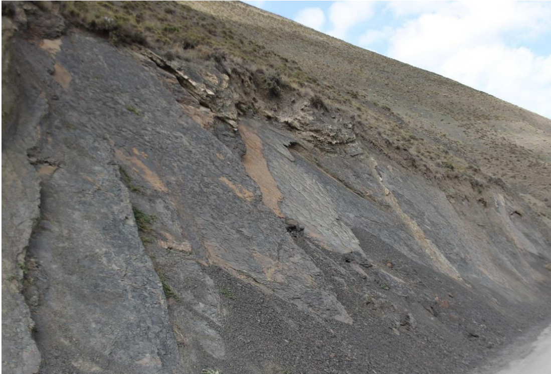
Photo 29: Many thin and easily breakable layers of the Middle Jurassic slates are responsible for their high natural erodibility. Here at the road between Bostankesh and Khinalig, note also the dominant thorn cushions of the genus Astracantha , which help stabilising these southern slopes with their deep roots (S. Hirschelmann).
