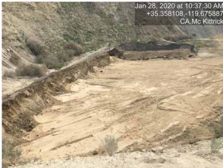
Figure 6: A cleaned-up oil/water surface expression in Cymric oil field, Kern County 2019. A berm and netting remain as a precaution (upper right) to contain any further oil and keep birds and animals out (CalGEM 2020).
