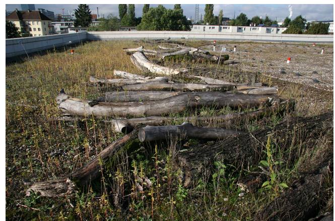
Fig. 7: School building Schoren, Basel, a green roof with a mixture of sandy gravel, compost, lava-pumice and wood, constructed in 2017. The site where Robertus mediterraneus was found for the first time north of the Alps (Photo: Stephan Brenneisen)
