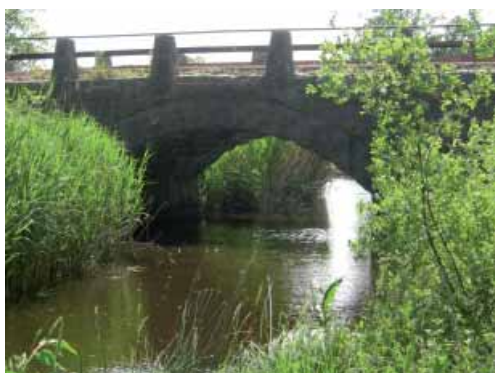
An old stone vault bridge crosses the Vieryd River where it meets the sea.
