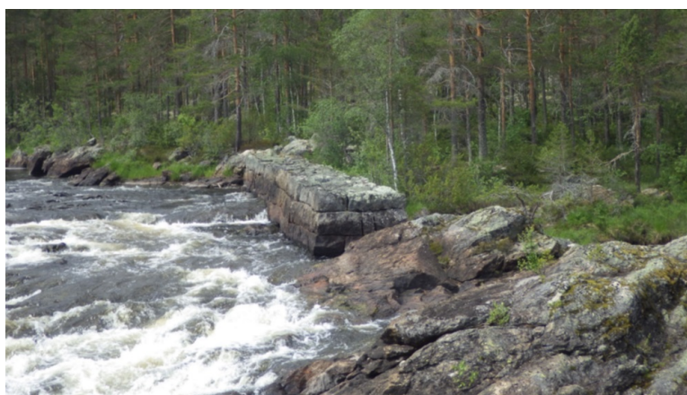
Figure 10.3: Historical remains of the log-driving epoch include built-up banks along the river. The picture shows a particularly substantial stone banking at the Hylströmmen rapids. Photography: Anders Persson/Linda Jonsson
